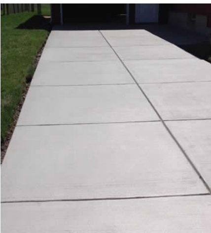
Broom Finished Concrete
